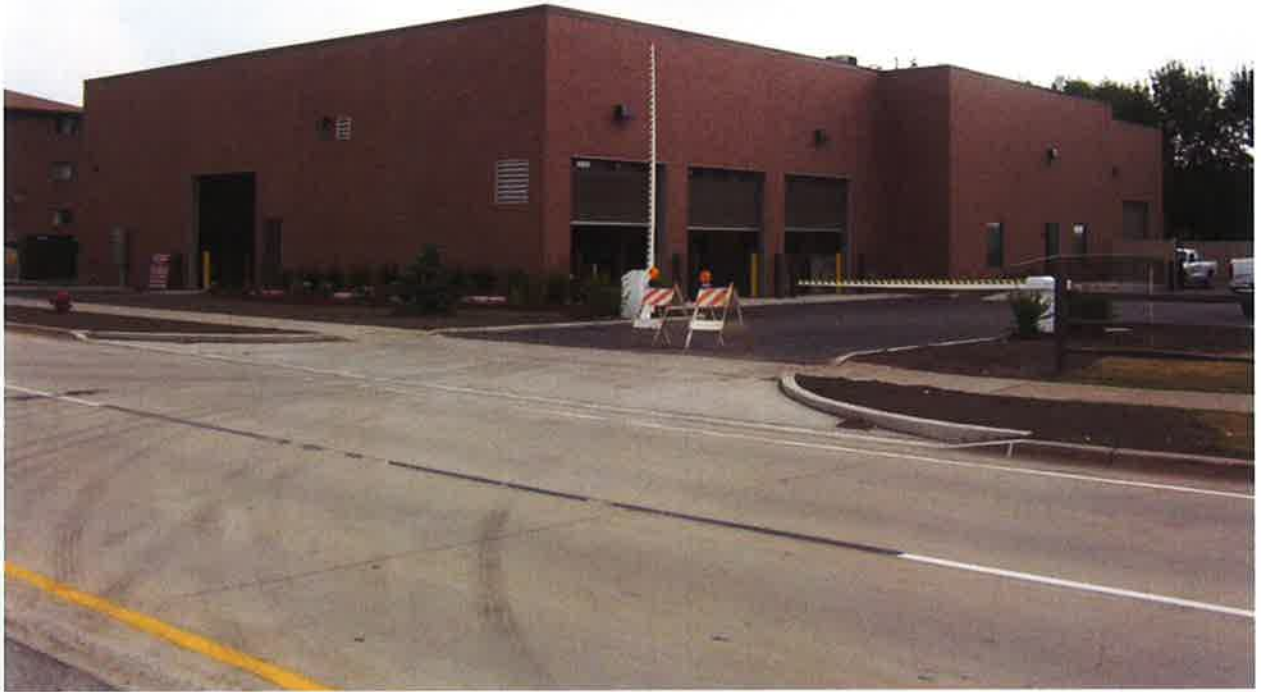
Tinley Park Park District Maintenance Facility
