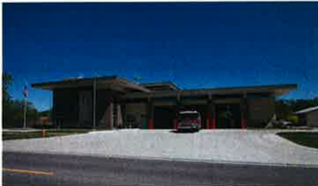
Mount Prospect Fire Station Mount Prospect, Illinois
