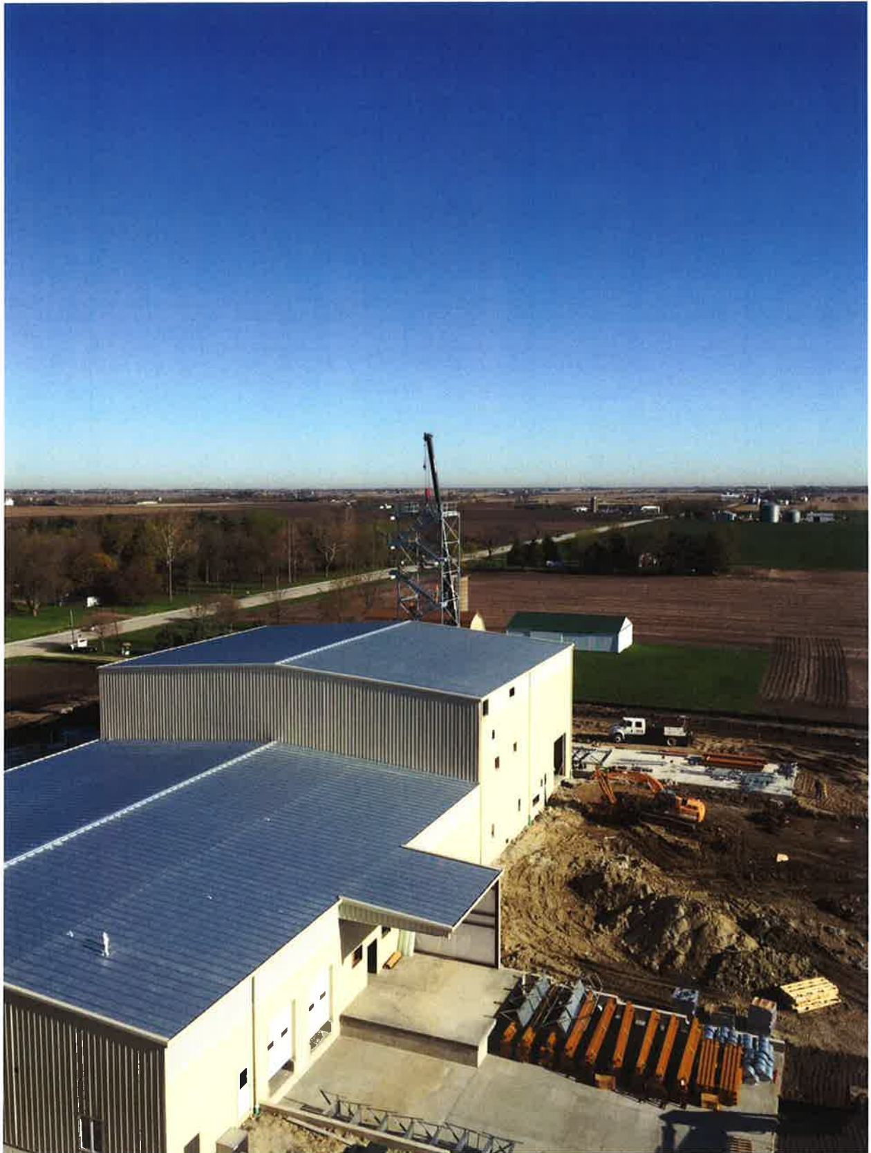
The Scoular Company- The largest soybean cleansing facility in North America with complete automation.
